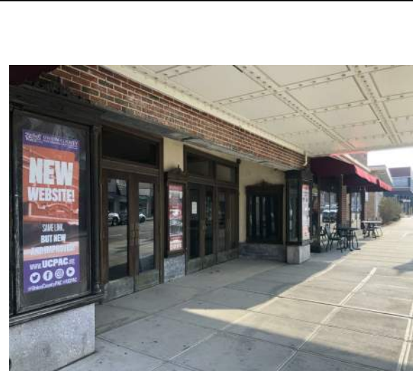
1 PHOTO DETAIL 01 OVERALL VIEW OF EXTERIOR
